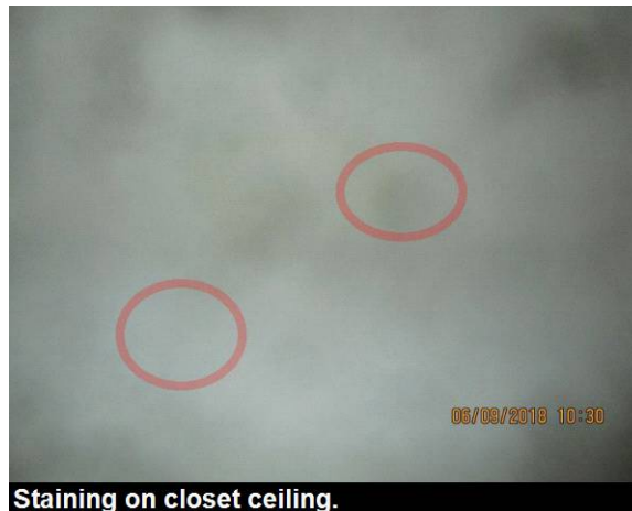
Staining on closet ceiling.
