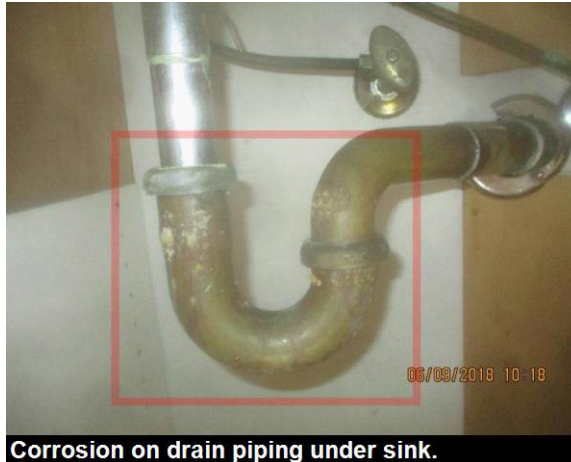
Corrosion on drain piping under sink.
