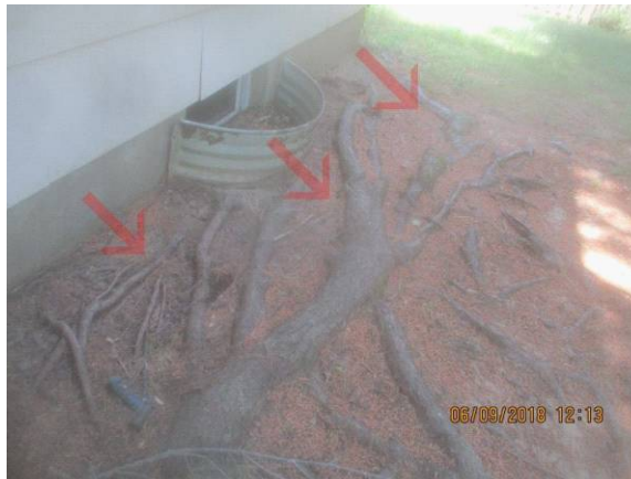
Tree roots along rear foundation wall.
