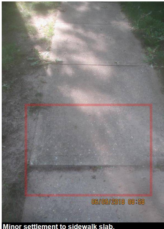
Minor settlement to sidewalk slab.
