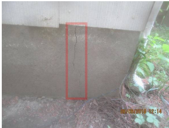
Vertical crack in rear foundation wall.
