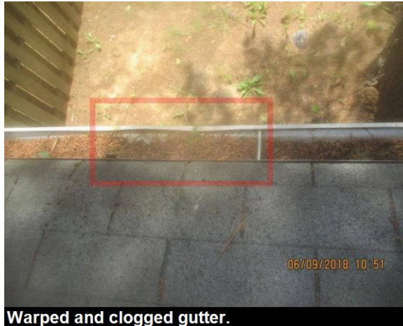
Warped and clogged gutter.
