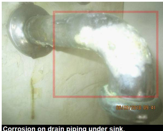
Corrosion on drain piping under sink.
