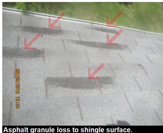
Damaged shingles at upper left rear roof.
