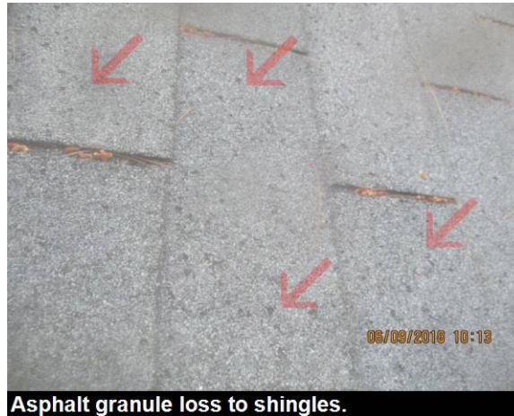
Asphalt granule loss to shingles.
