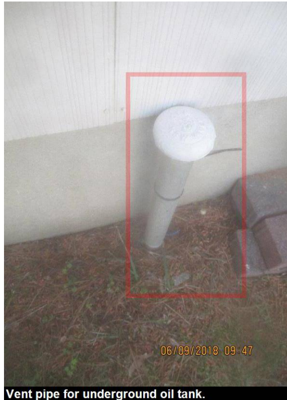
Vent pipe for underground oil tank.
