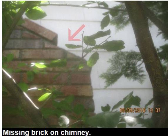
Missing brick on chimney.
