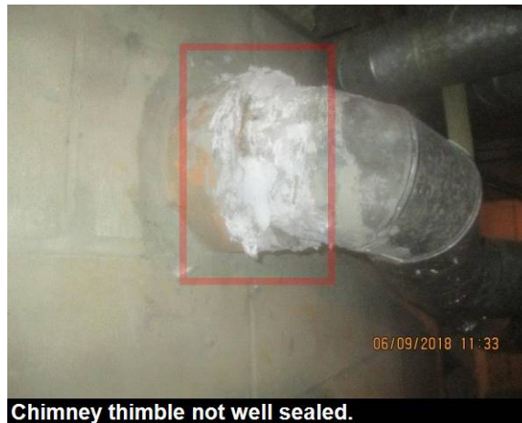
Chimney thimble not well sealed.
