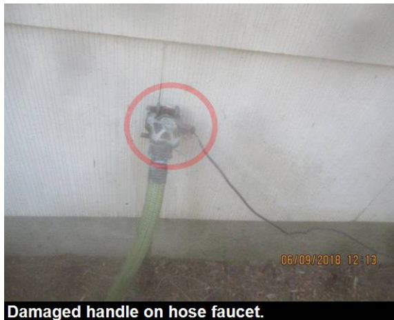
Damaged handle on hose faucet.
