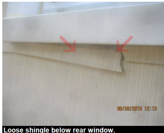
Loose shingle below rear window.
