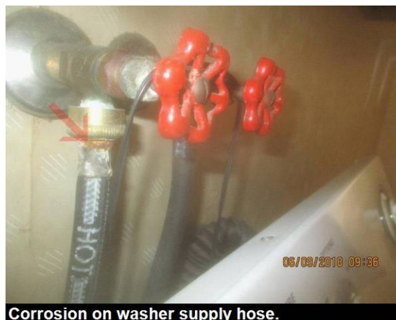
Corrosion on washer supply hose.
