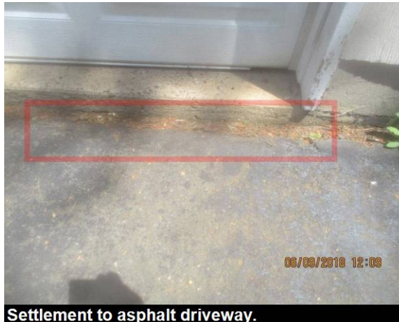
Settlement to asphalt driveway.
