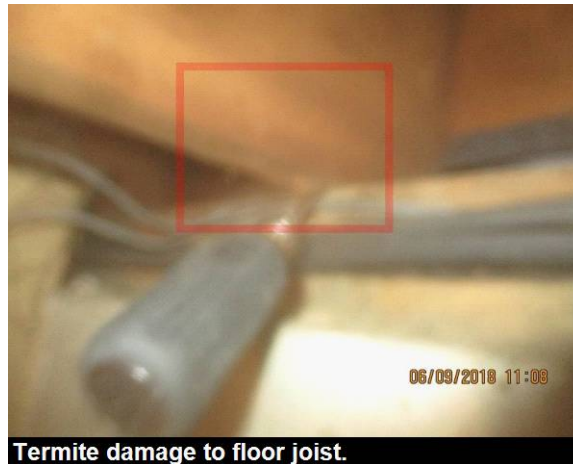
Termite damage to floor joist.
