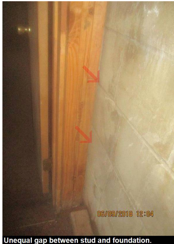
Unequal gap between stud and foundation.
