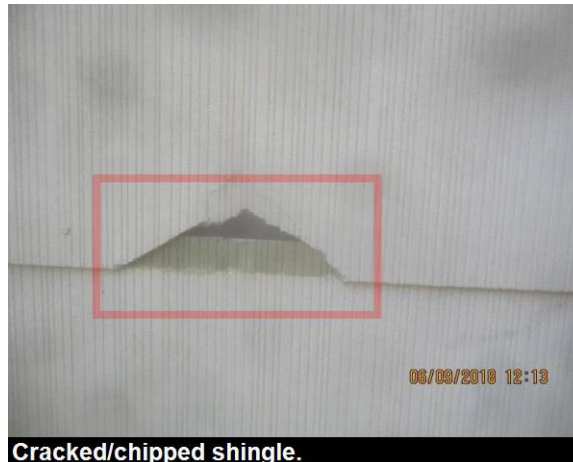
Cracked/chipped shingle.
