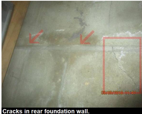
Cracks in rear foundation wall.
