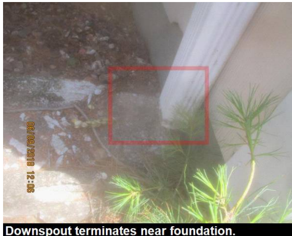
Downspout terminates near foundation.
