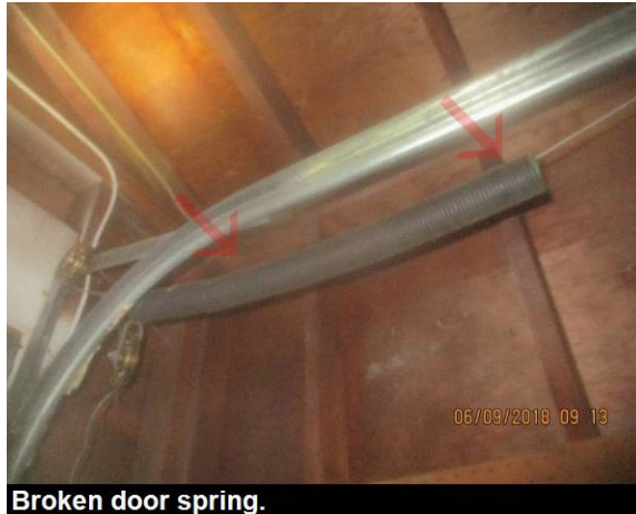
Broken door spring.
