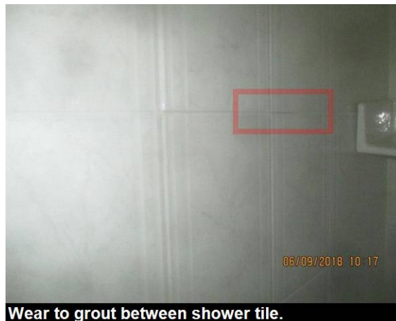
Wear to grout between shower tile.
