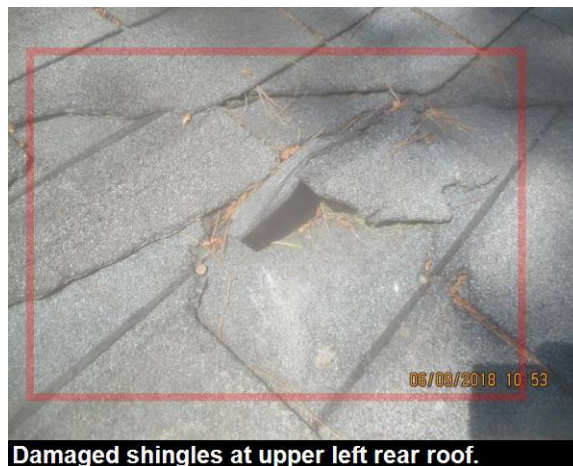
Damaged shingles at upper left rear roof.
