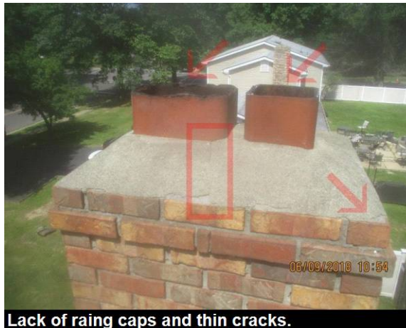
Lack of raing caps and thin cracks.
