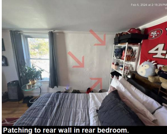
Patching to rear wall in rear bedroom.
