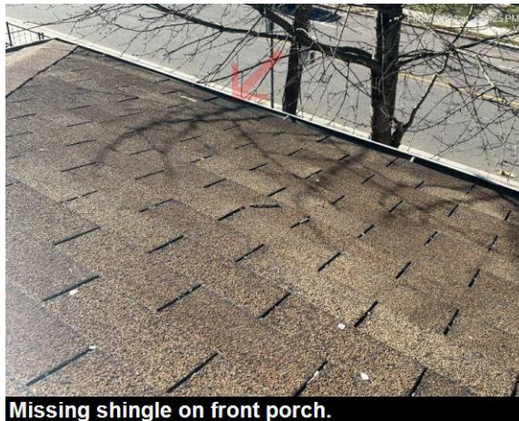
Missing shingle on front porch.
