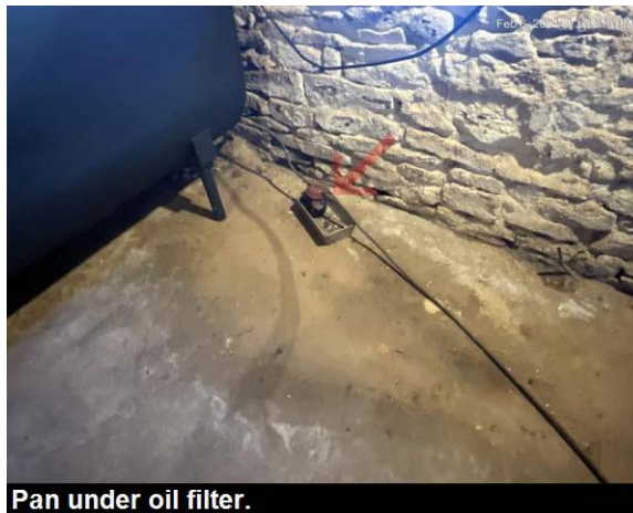
Pan under oil filter.
