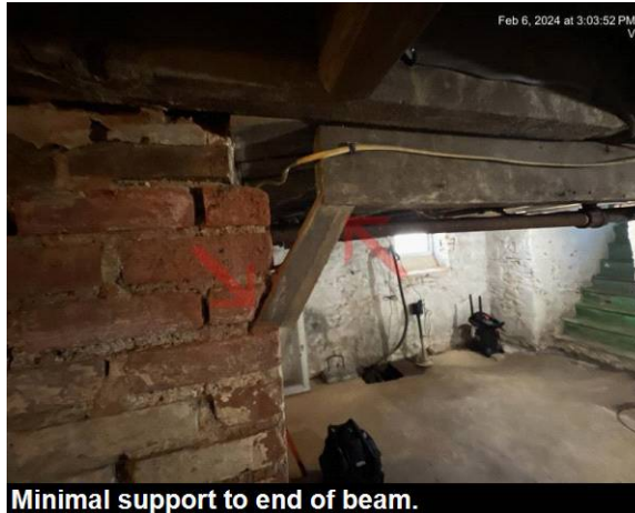
Minimal support to end of beam.
