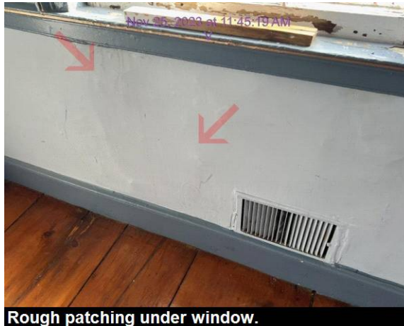
Rough patching under window.
