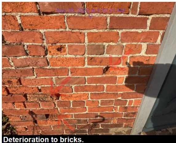
Deterioration to bricks.
