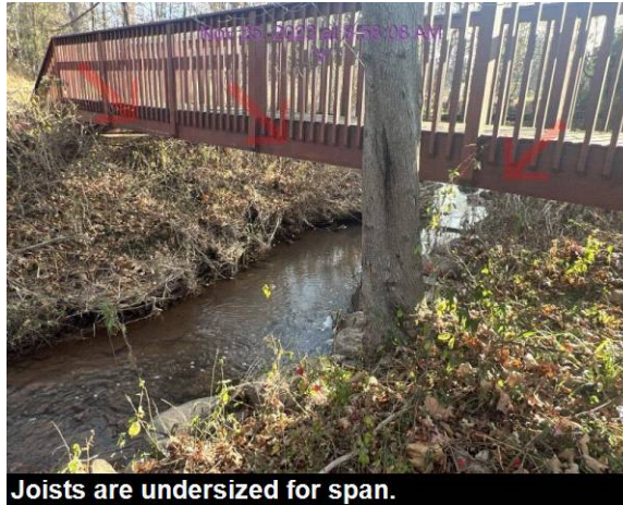
Joists are undersized for span.
