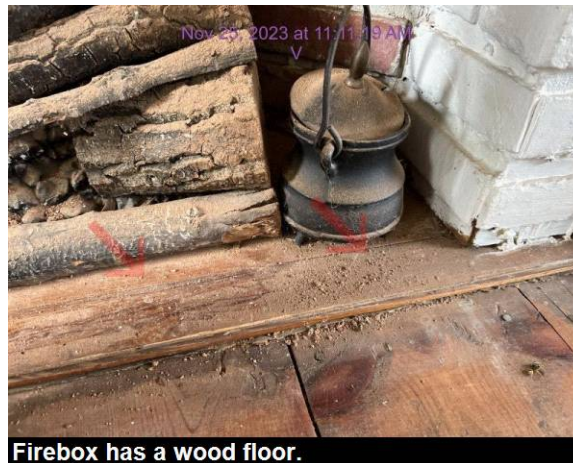
Firebox has a wood floor.
