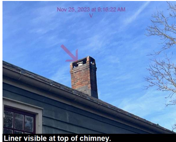
Liner visible at top of chimney.
