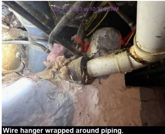
Wire hanger wrapped around piping.
