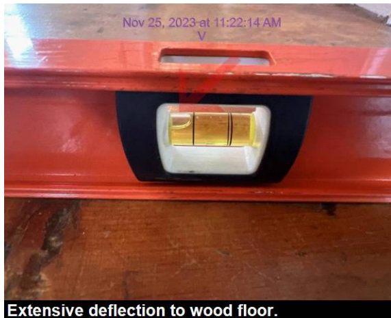
Extensive deflection to wood floor.
