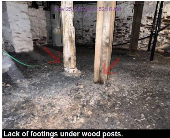
Lack of footings under wood posts.
