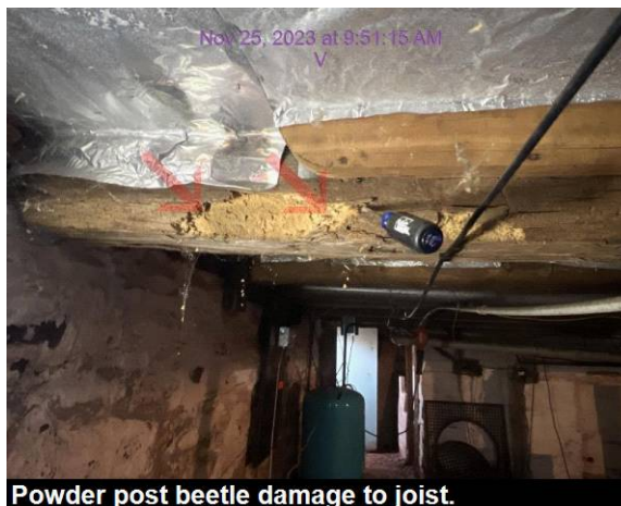
Powder post beetle damage to joist.
