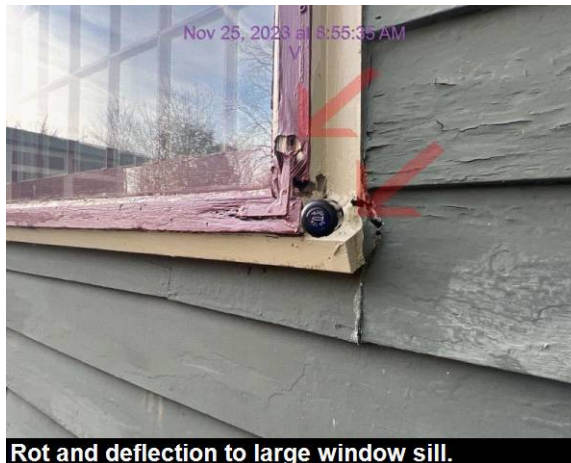
Rot and deflection to large window sill.
