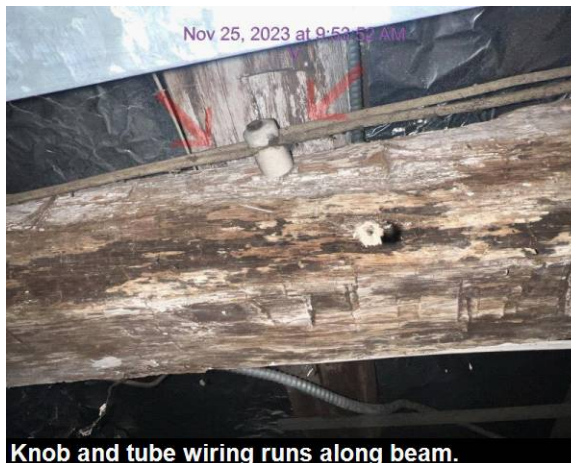
Knob and tube wiring runs along beam.
