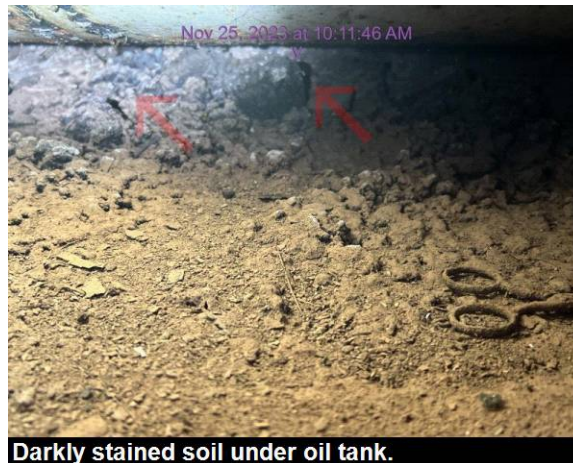
Darkly stained soil under oil tank.
