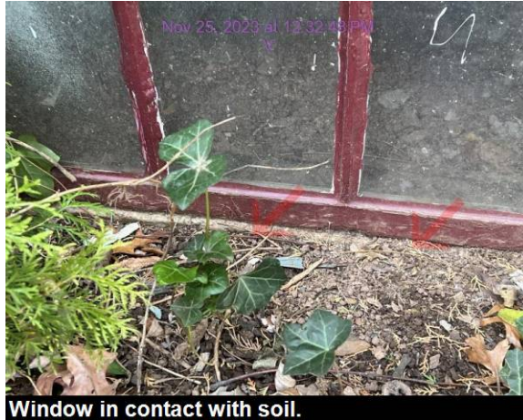
Window in contact with soil.
