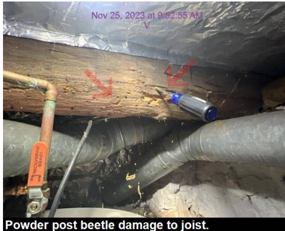
Powder post beetle damage to joist.
