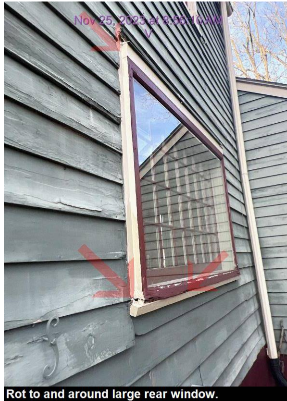
Rot to and around large rear window.
