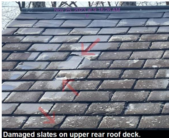
Damaged slates on upper rear roof deck.
