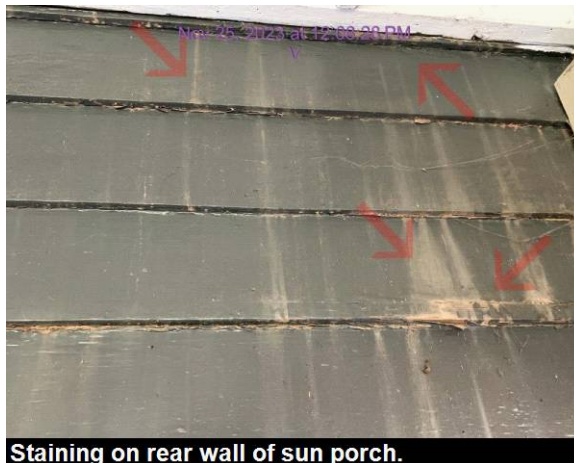
Staining on rear wall of sun porch.
