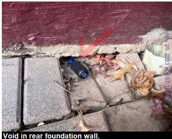
Void in rear foundation wall.
