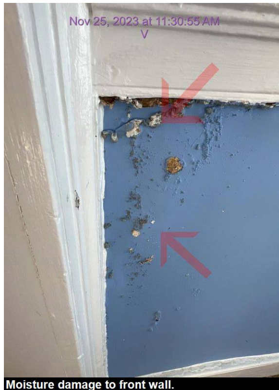
Moisture damage to front wall.
